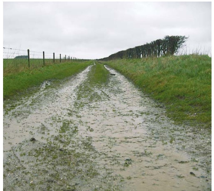
Figure 17. Surface run-off can wash soil onto adjacent field tracks or roads
